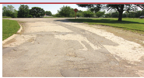
DAMAGED CONCRETE ROAD
